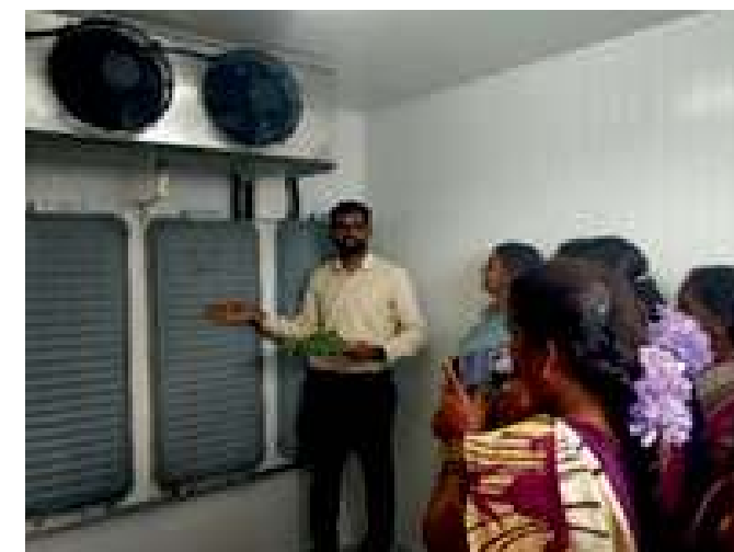
Electrical battery free: Installed PCM plates act as thermal batteries.
