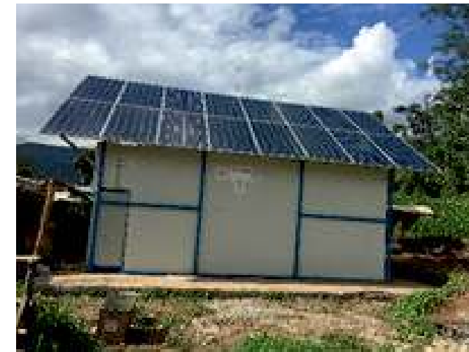
5 MT PCM based cold room (3 MT and other customized solutions also available).
