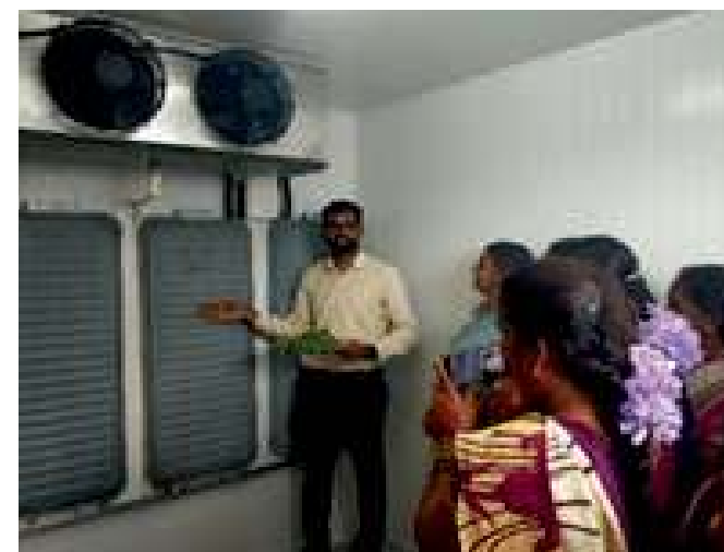
Electrical battery free: Installed PCM plates act as thermal batteries.
